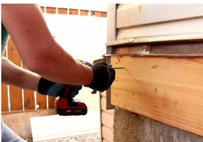
1. Determine the desired finish height of the deck. Then determine the thickness of the stone, the membrane, and the plywood; these typically add up to 1 3/4". This is a good height for the ledger board. It is not critical that the ledger board be specifically at this height as you can adjust the final height of the joists.
