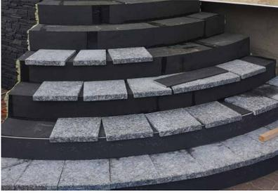
1. Install all the Tanzite edge and corner stones. First mark the location of pre-drilled holes in the Tanzite stone onto the concrete surface.
