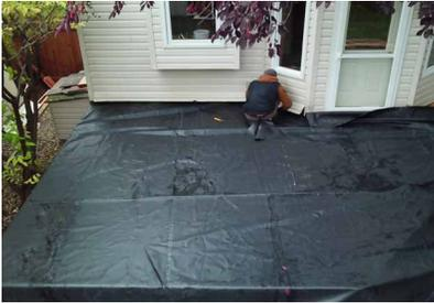
2. Place a full piece of EPDM roofing membrane of the wooden structure and fit into place. Do not cut.
