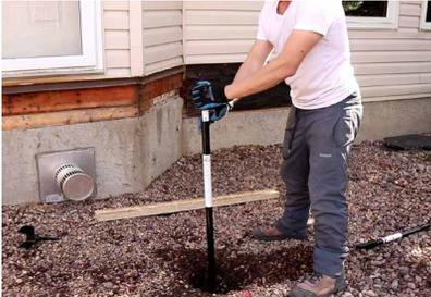
1. Determine where each pile is to be located and ensure there are no buried hazards, like a gas line, where you will put each pile.
