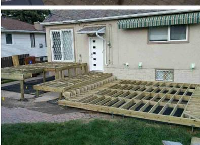
1. Determine the desired finish height of the deck. Then determine the thickness of the stone, the membrane, and the plywood; these typically add up to  $1\frac{3}{4}$ "
