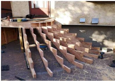
3. Then divide total height by the number of rises needed to determine the rise height (Example 48" divided by 7 is  $6\frac{7}{8}$ "). The run should always be  $10\frac{1}{2}$ " to work perfectly for the stone.
