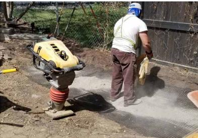
1. Cover the base material with fine rock material. (Example: sand)
