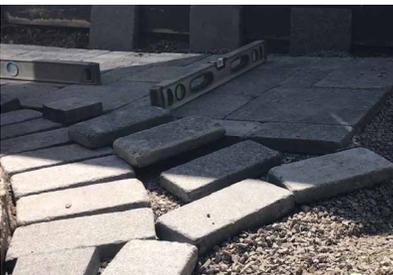
1. Install a Snap Edging (or similar) plastic edge border around the perimeter. The top edge of the plastic should only extend above the prepared base 3/4”.
