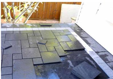
1. First lay the edge stones along the house to ensure the membrane is not tensioned. Then again ensure the membrane is flat with no wrinkles
