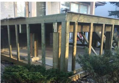
1. Install a vertical stud to the back of the joist/rim board every 2' on centre all around the deck.
